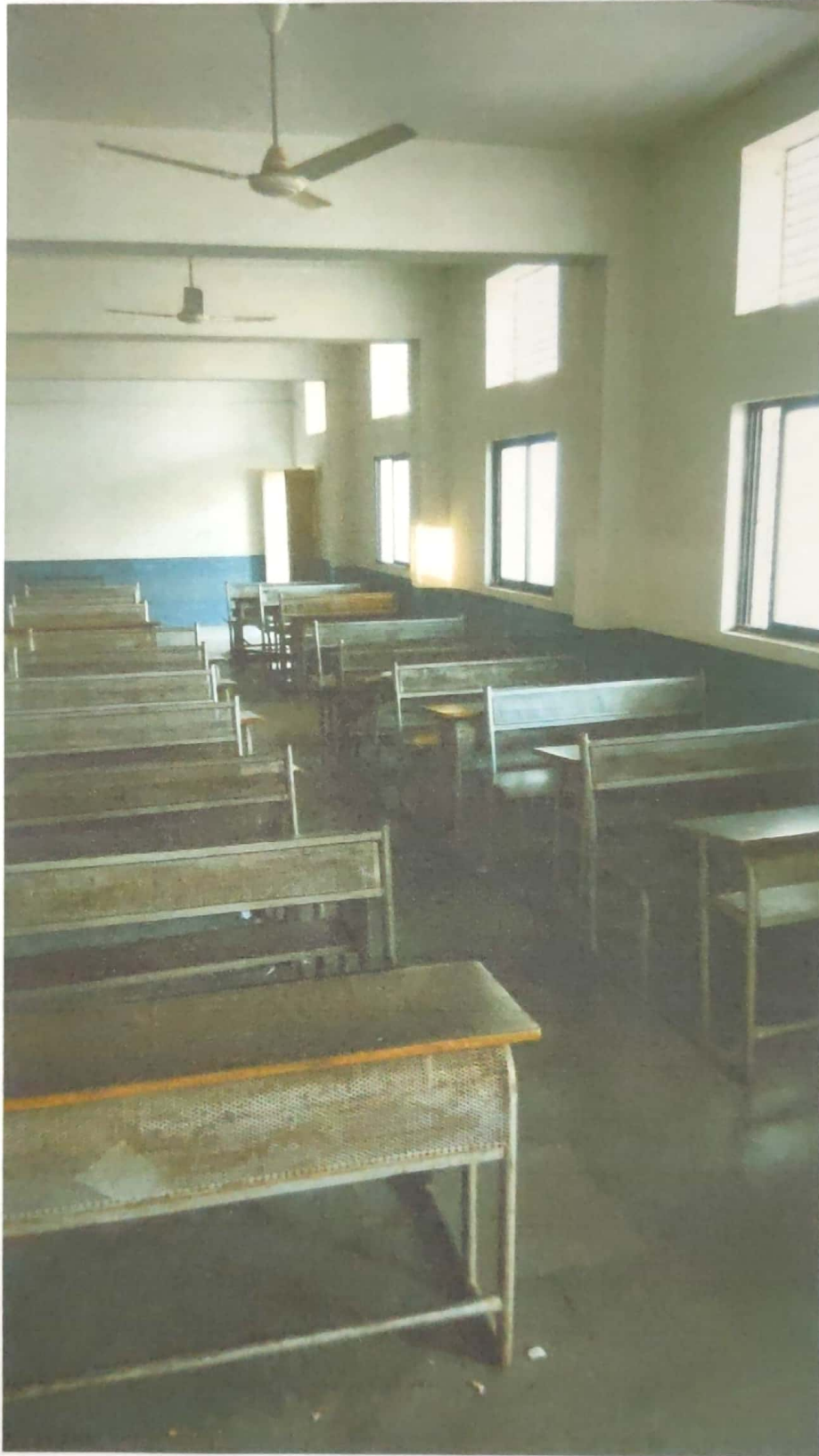
Photo 16 Classroom's ventilation is natural draft through windows
