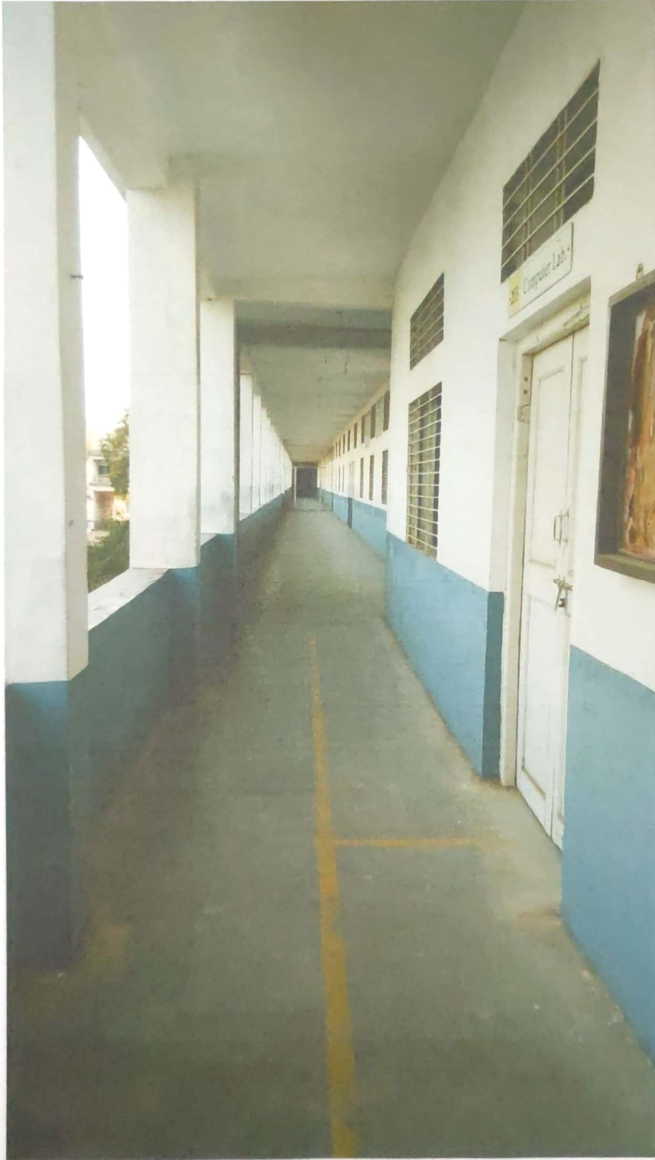
Photo 10 Well Ventilated corridor
